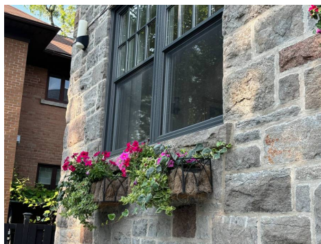
Back of building — 435 Laird
